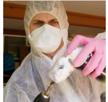
Preparing to drill hole in ceiling.
